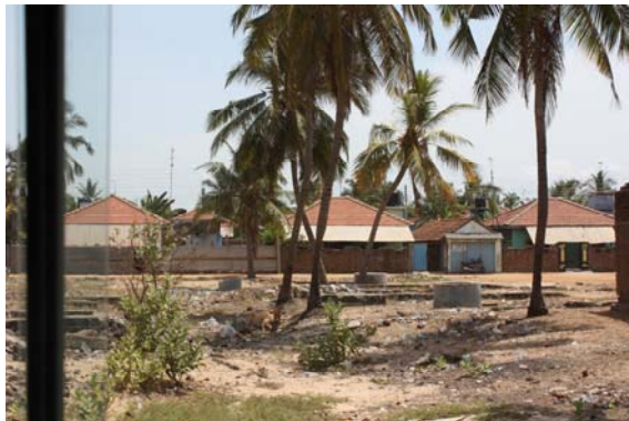
Kalmunai (tsunami damage in foreground): from this ....
